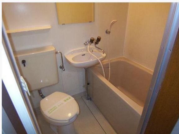
Example of a unit bathroom with shower, bath tub, sink, and toilet all in the same space. This is a common layout for studio apartments. Newer buildings tend to split up the toilet and washroom spaces, even in studio apartments. Photo: Real Estate Japan
