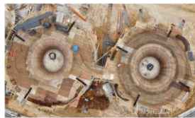
Flat slab & Concrete shell 3D formwork
